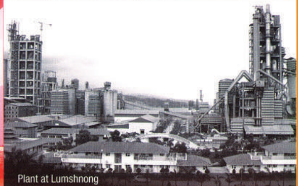
Plant at Lumshnong
